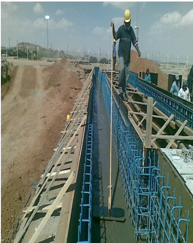
Concrete Trenches in Progress
