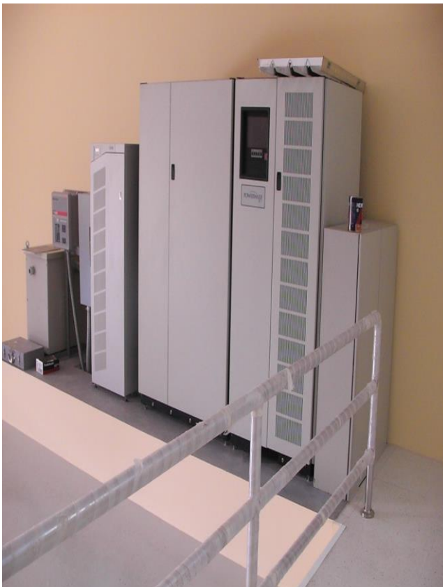
Frequency Converter and UPS for Simulators
