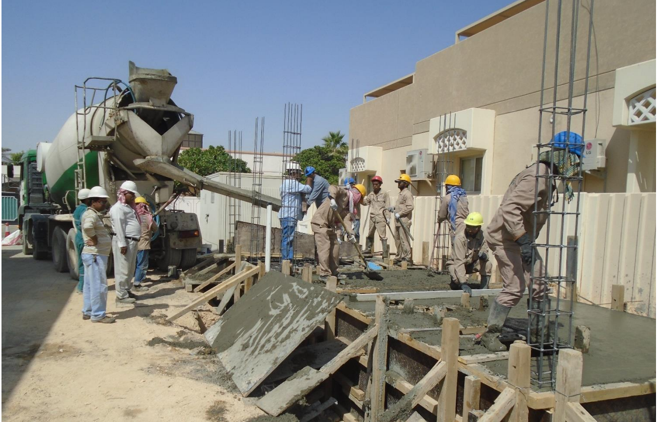
Foundation Work of Transformer, Eskan Village, Riyadh
