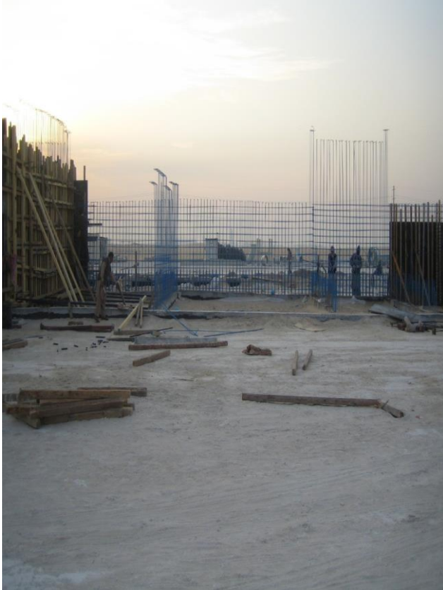
Concrete walls for Industrial Plant
