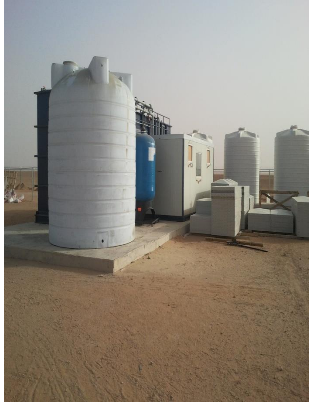
STP Installation for Temporary facilities
