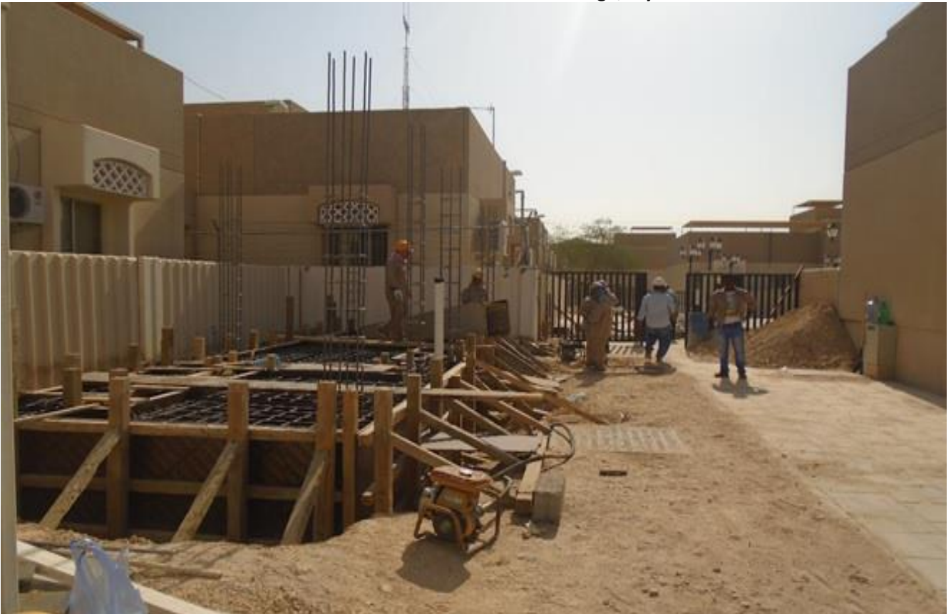
Foundation Work of Transformer, Eskan Village, Riyadh
