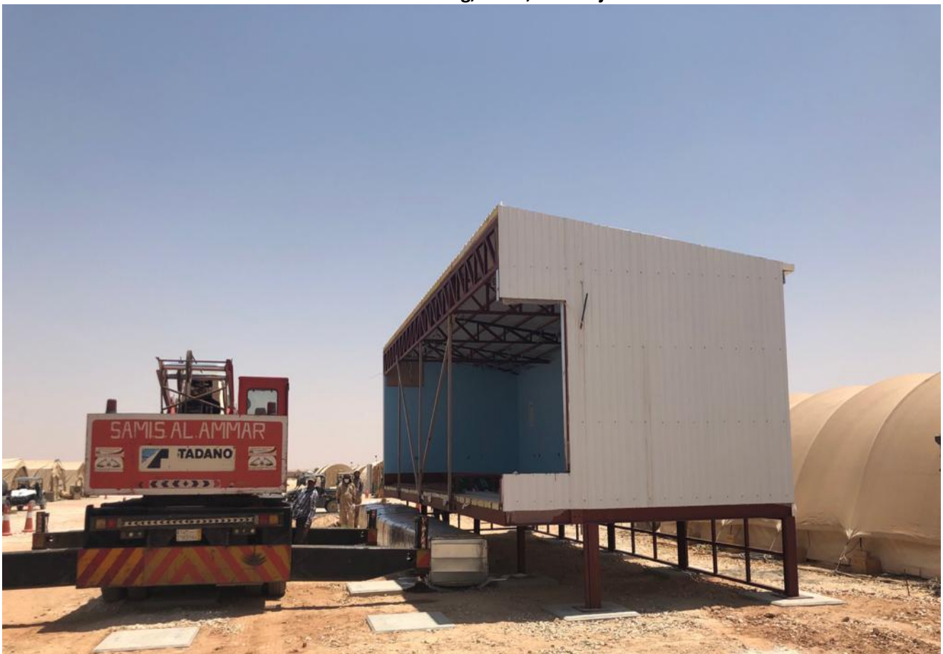
NCC Trailer Building, PSAB, Al Kharj-KSA
