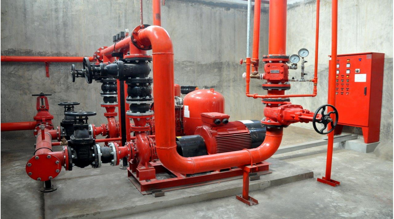
Fire Fighting and Fire Suppression Work (FM200), Riyadh Metro Project, KSA
