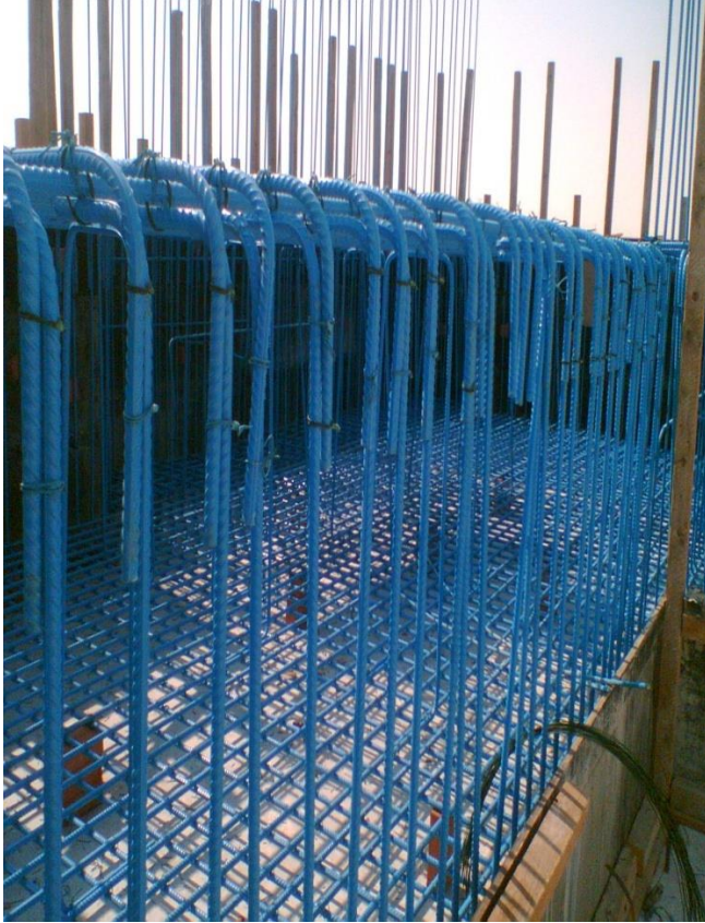
Foundation work for Sabic Hadeed
