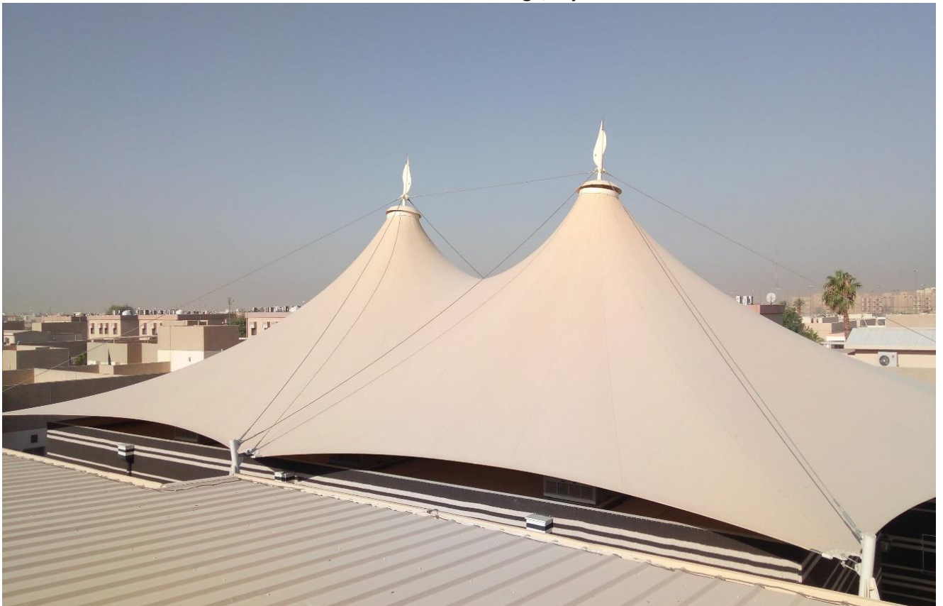
Canopy – OCCF Project – Eskin Village, Riyadh
