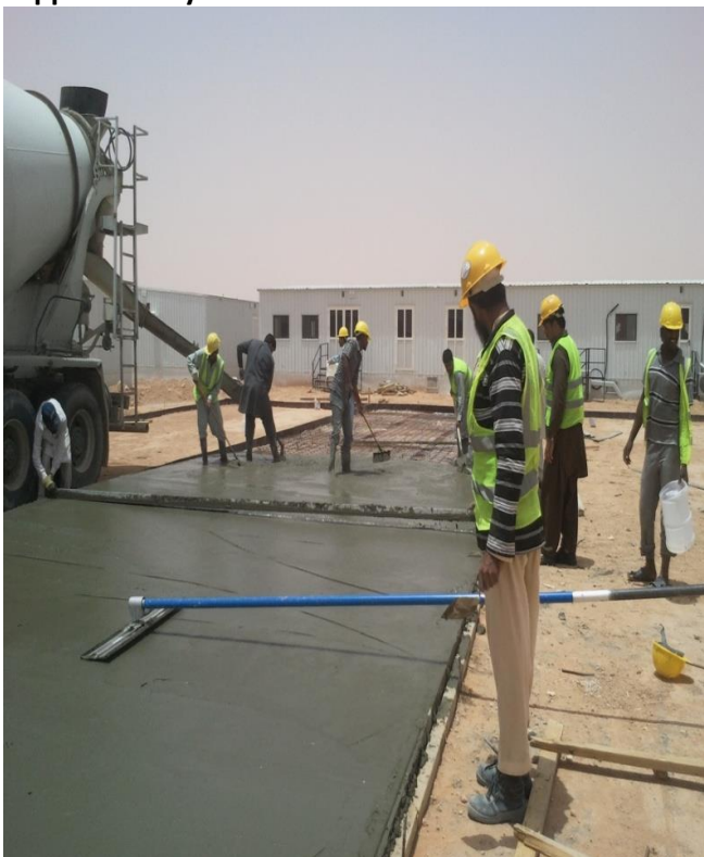
Concrete slab pouring and tooling
