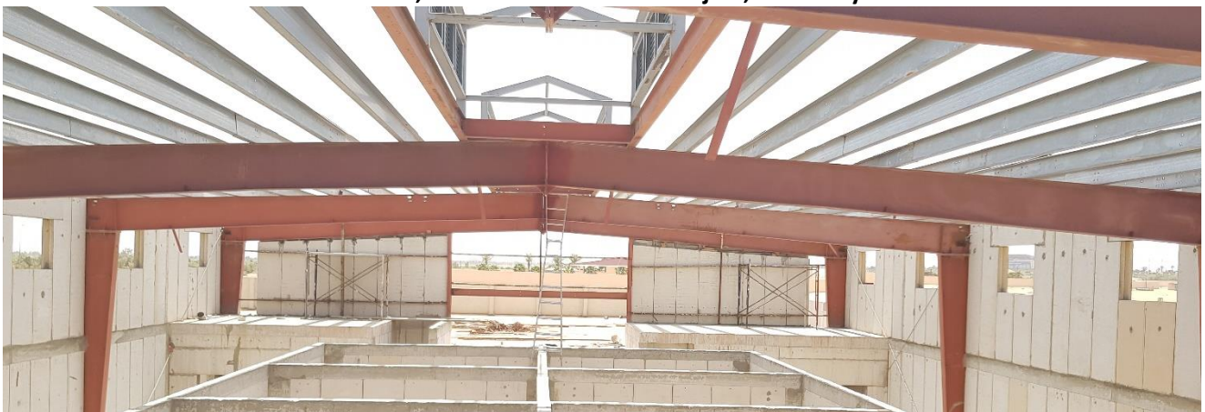
Trainer's Villa, Precast Soleed Panel Project, Janadariyah-KSA
