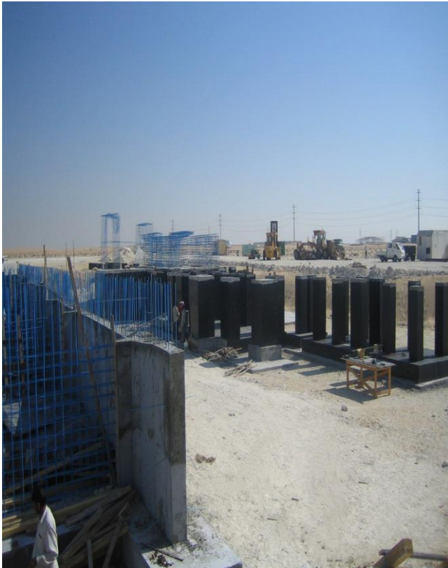
Foundation work for Steel Recycling Plant
