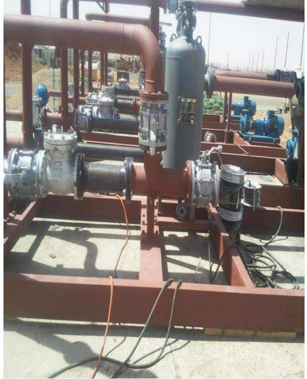
Fabrication of pump skid for offloading. fuel at SEC Power Plant
