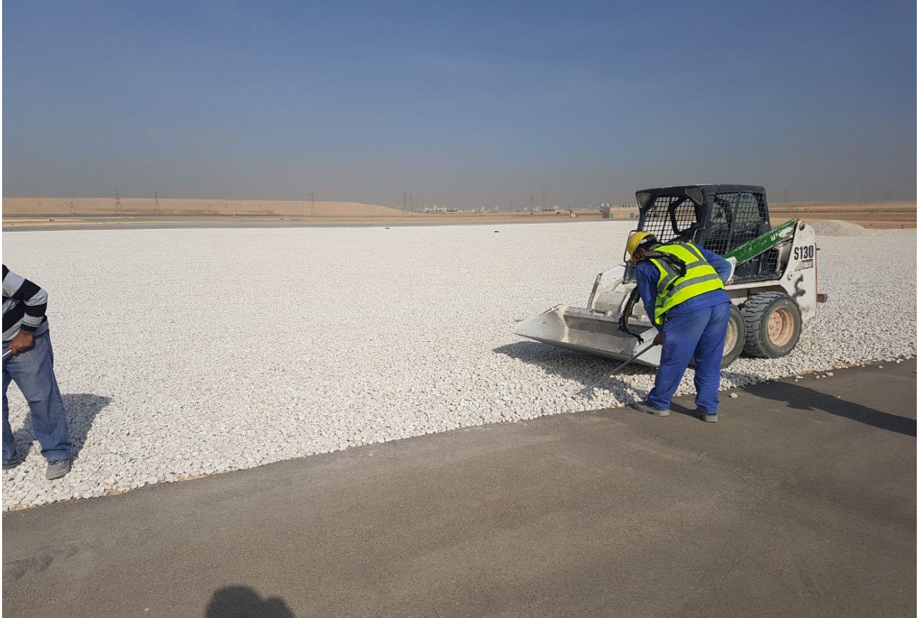
Supply and installation of Crushed Aggregate, Airfield-KAA, Riyadh
