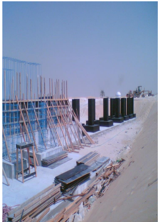
Foundation work for Steel Recycling Plant
