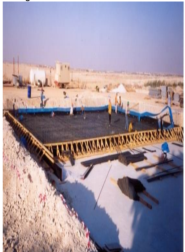
Form work for water tank in Progress
