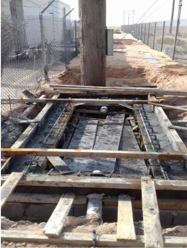
SCECO Project, Foundation of septic tank, Harfal Batin
