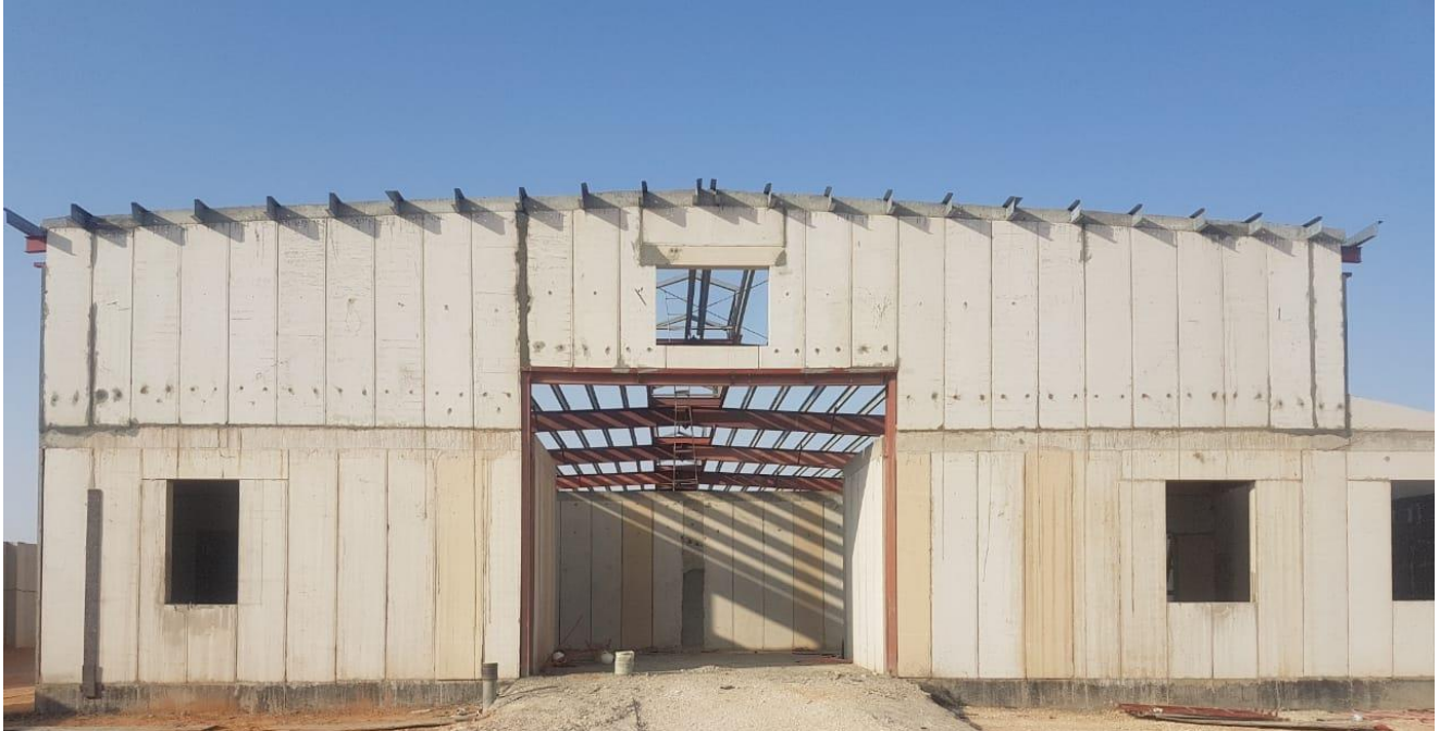
Trainer's Villa, Precast Soleed Panel Project, Janadariyah-KSA
