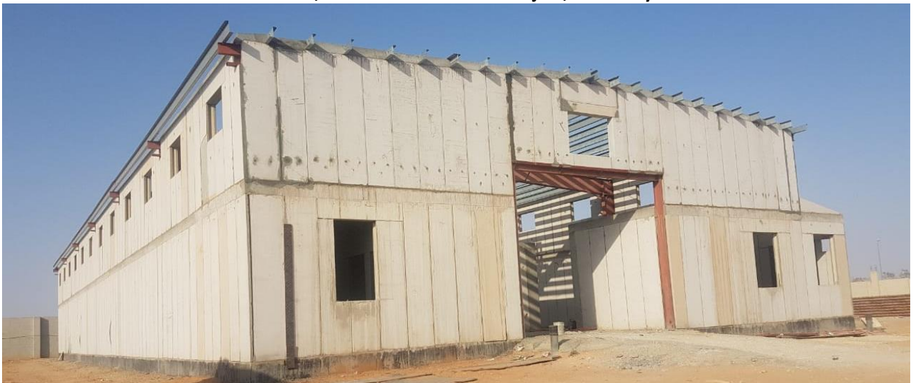
Trainer's Villa, Precast Soleed Panel Project, Janadariyah-KSA
