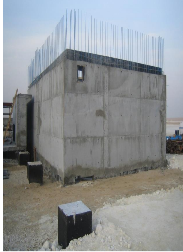
Explosion Proof Electrical Room
