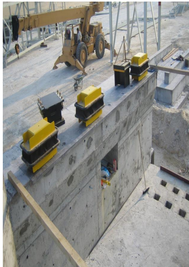
Concrete structure for Heavy crusher and AVMs
