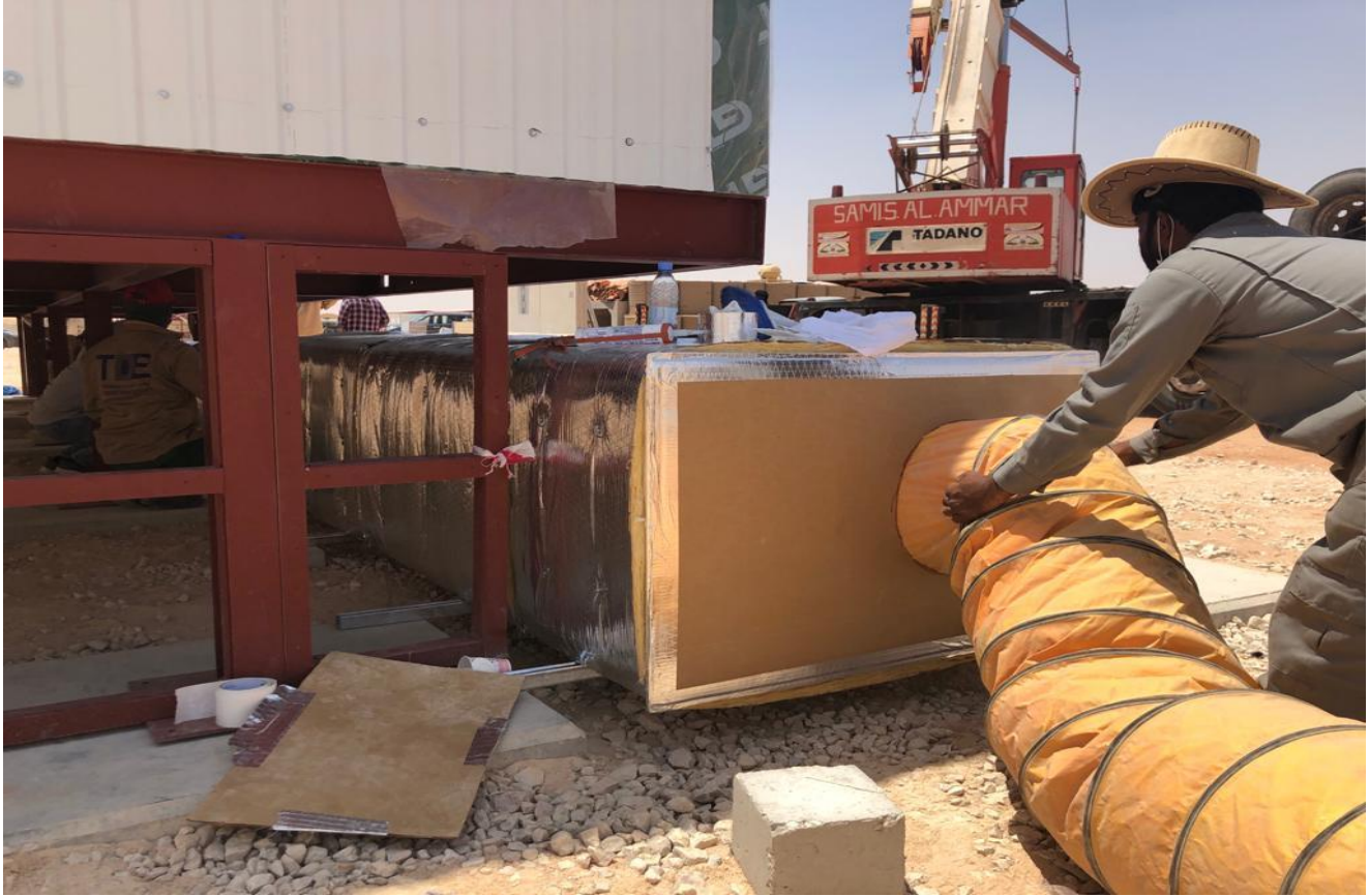
Installation of Flexible Ducts, NCC Trailer Building, PSAB, Al Kharj-KSA
