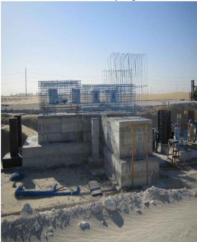
Foundation for Heavy machinery
