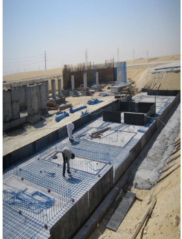
Foundation work for Steel Recycling Plant
