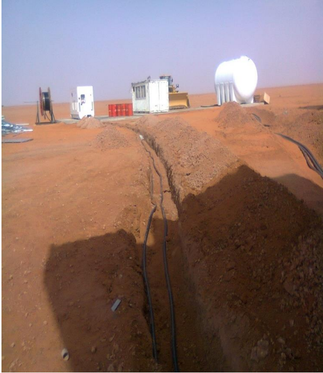
Cable Laying for Temporary facilities
