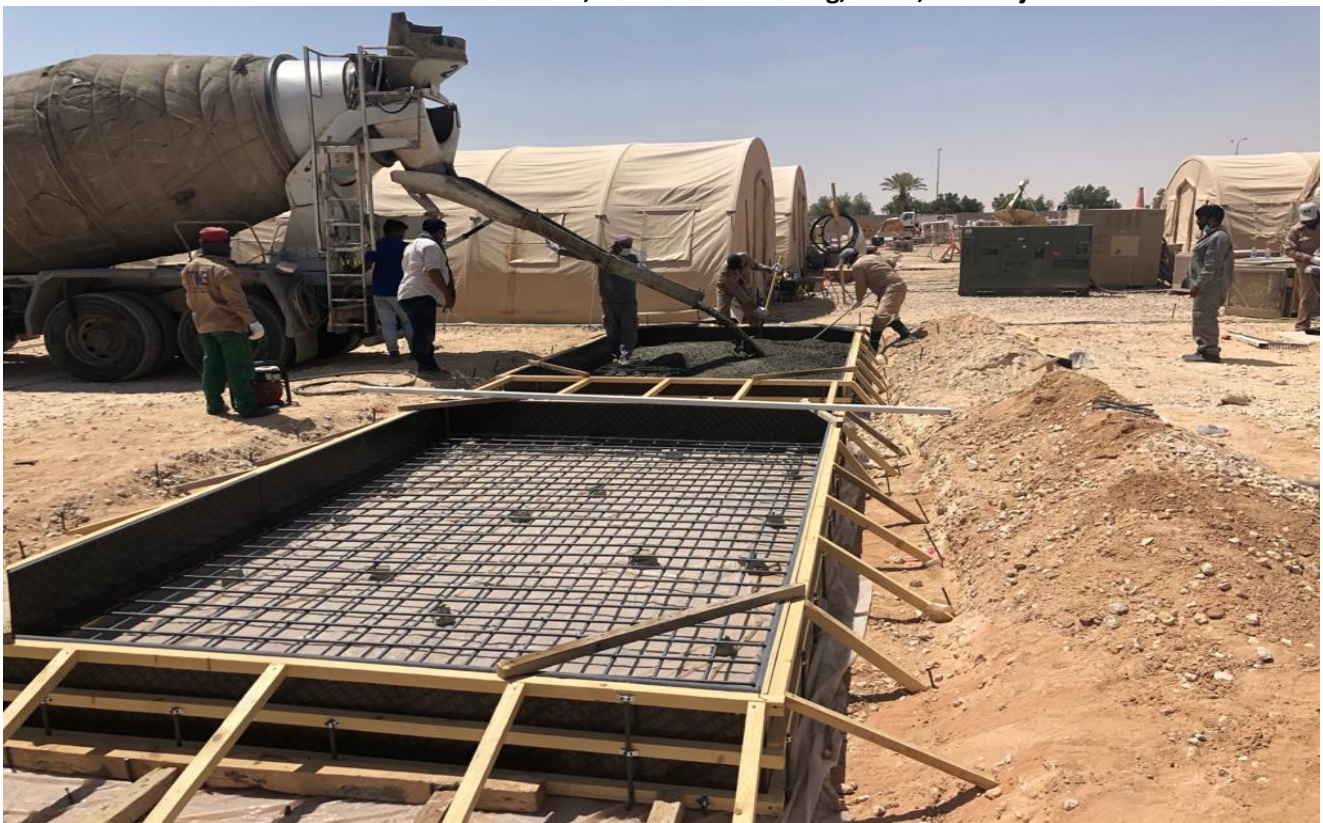
Construction of Concrete Pads for HVAC Units, NCC Trailer Building, PSAB, Al Kharj-KSA
