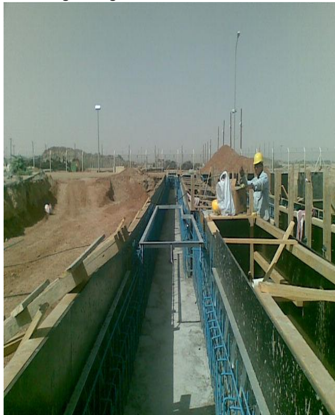
Fuel Pipe Trenches SEC Bisha
