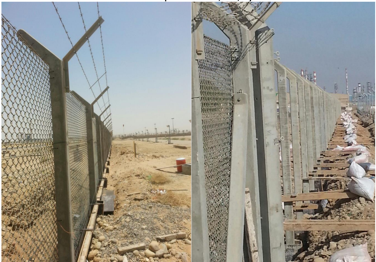
Construction of Chain Link Fence, Aramco Project, Dammam-KSA
