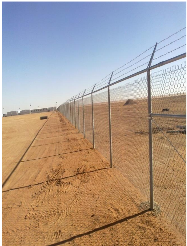
Chain-link fence Installation
