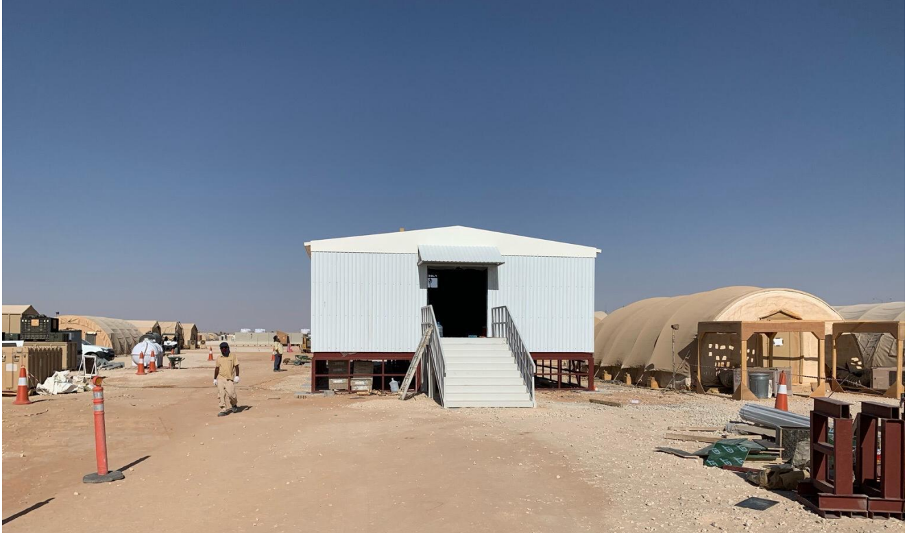
NCC Trailer Building, PSAB, Al Kharj-KSA
