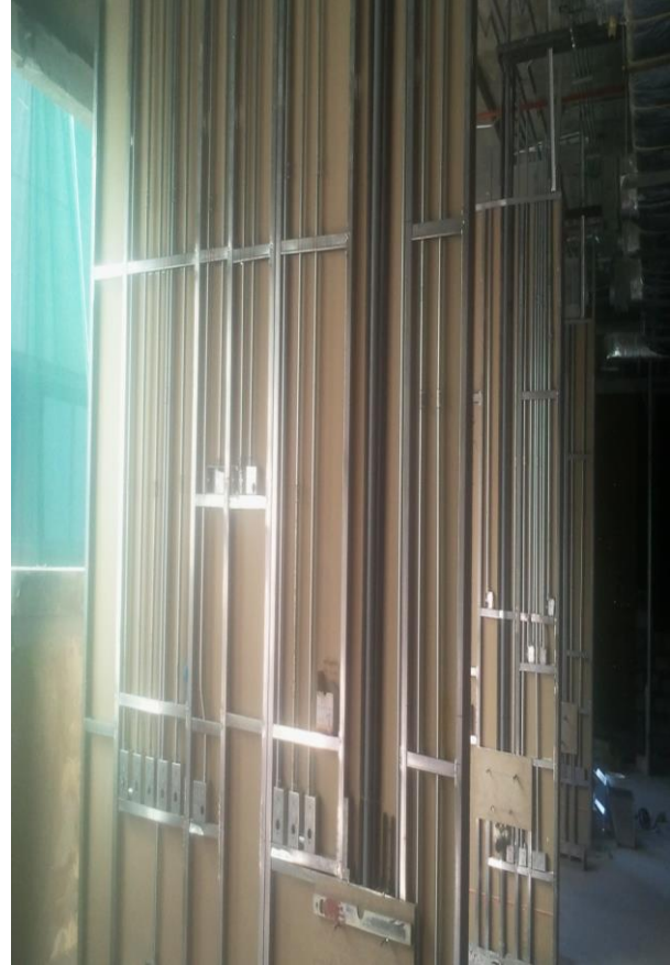
Partition works with rough-in electrical conduits for Hospital.
