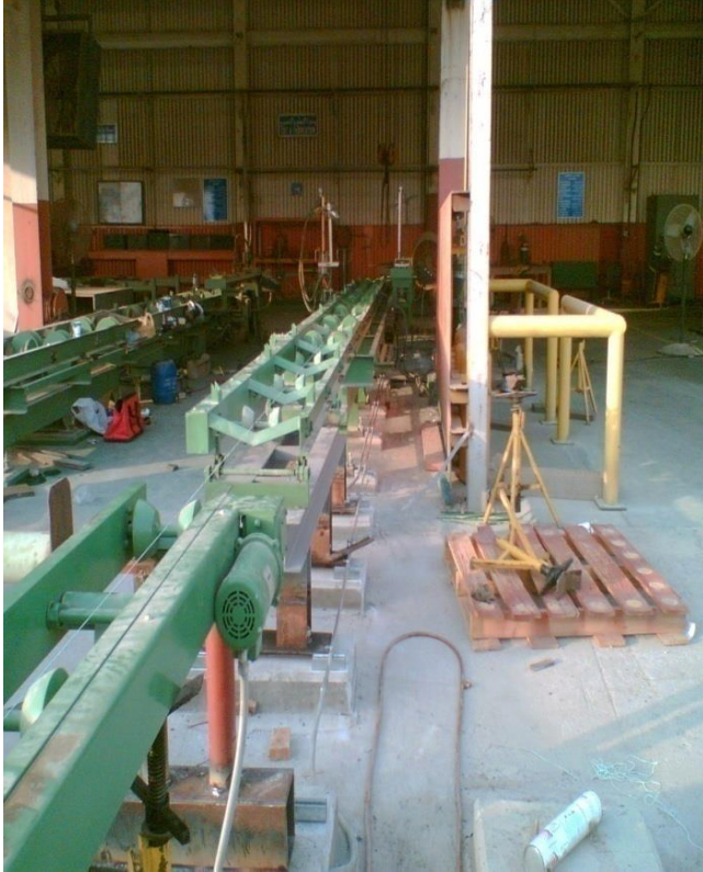
Foundation Work for Pantograph machines
