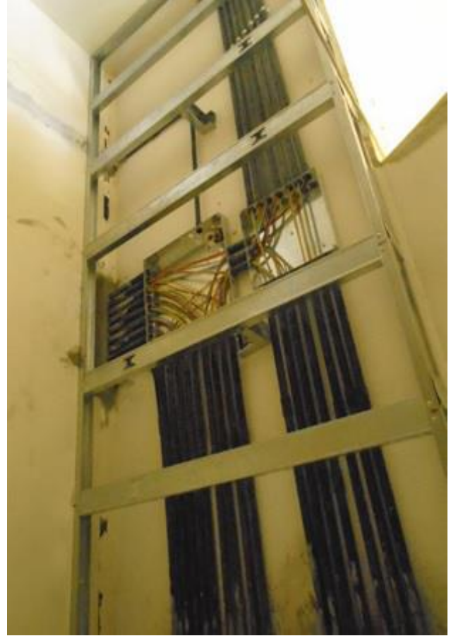
Cabling work, Eskan Village, Riyadh
