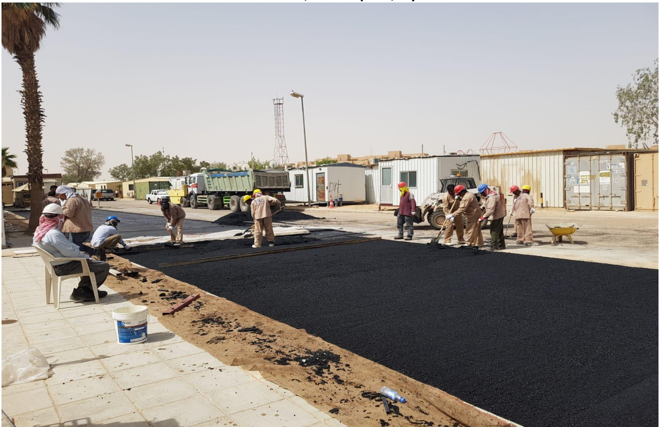
Road Construction at Eskin Village, Riyadh-KSA
