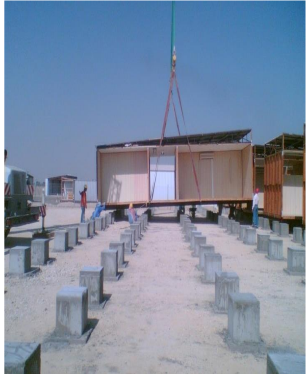
Portacabin Foundation works Temporary facilities
