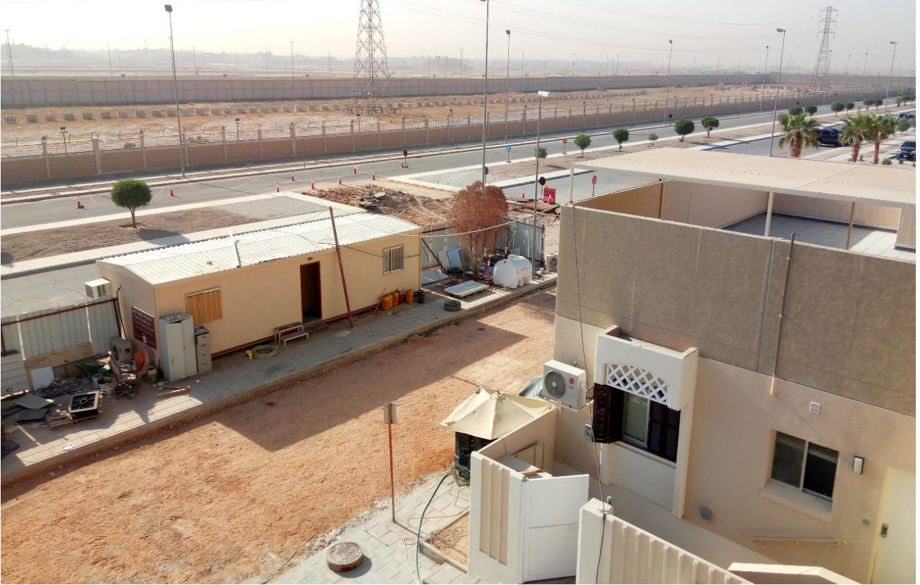
Renovation of Office Villas – Eskan Village, Riyadh
