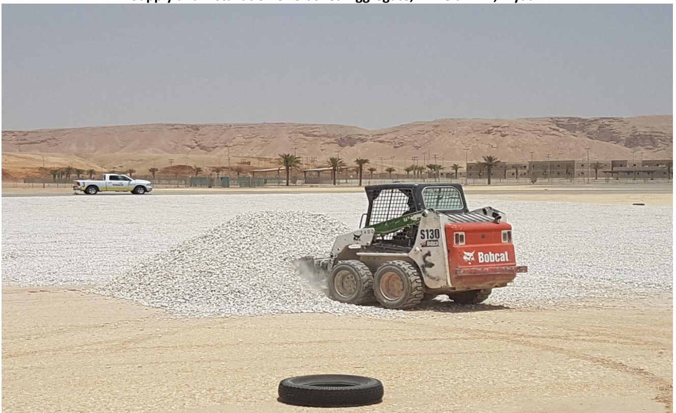
Supply and installation of Crushed Aggregate, Airfield-KAA, Riyadh
