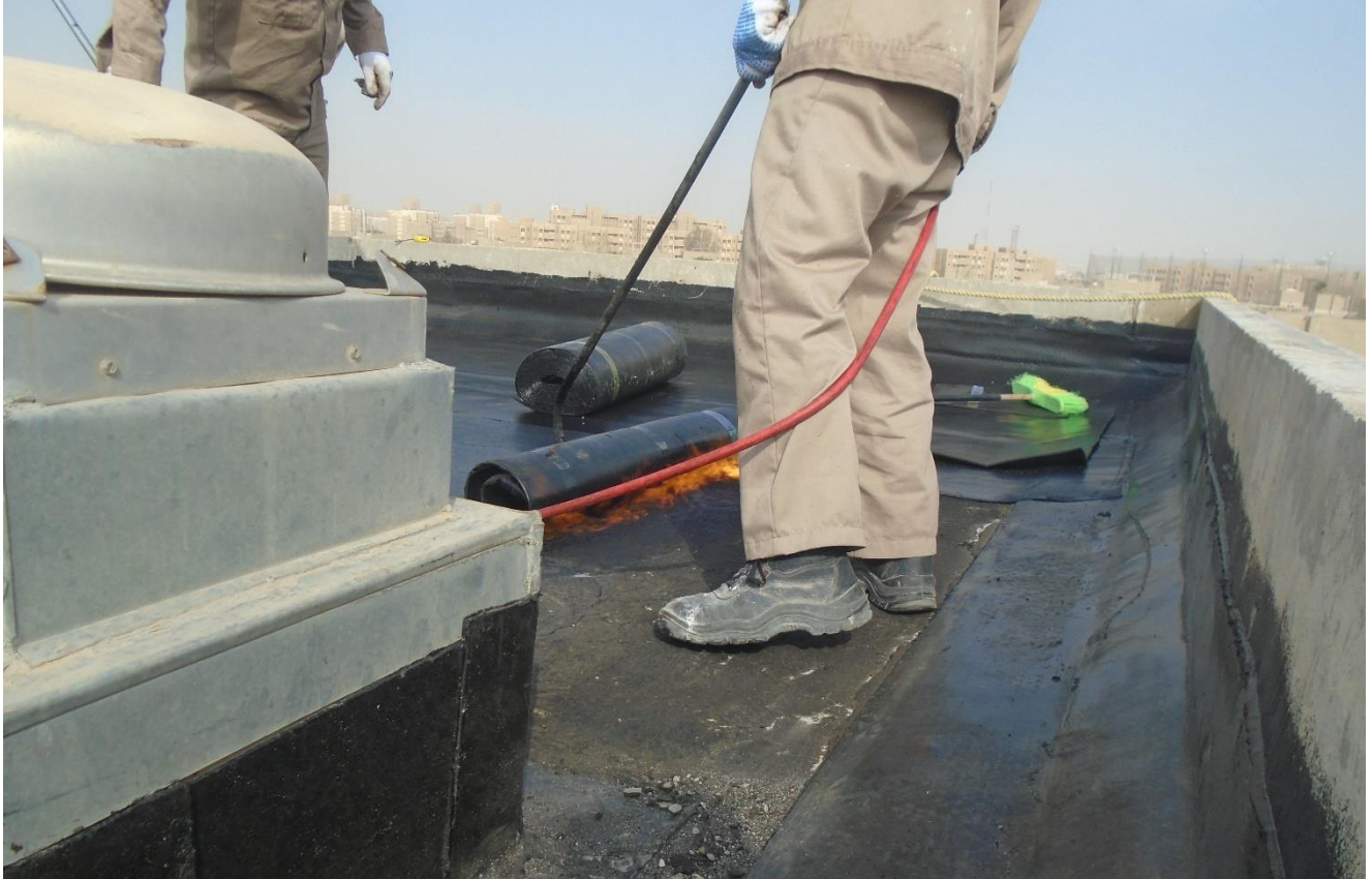
Water Proofing Membrane – Office Villas, Eskin Village, Riyadh
