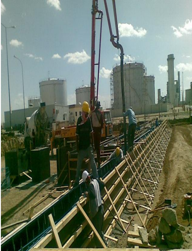
Concreting in Progress
