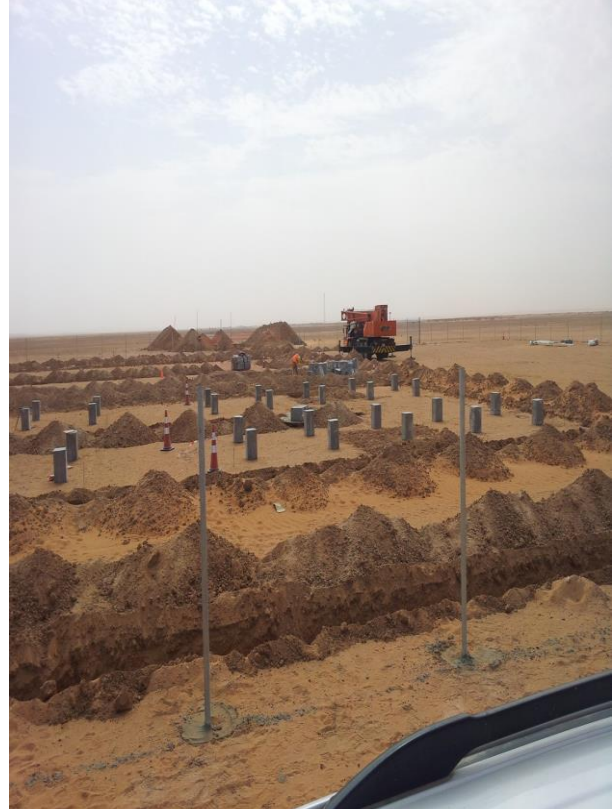
Fly Camp Ma'aden utility lines fence and building footings.
