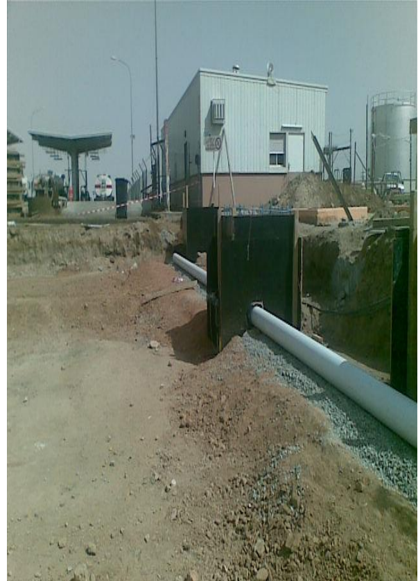
Fuel Drainage Line Installation
