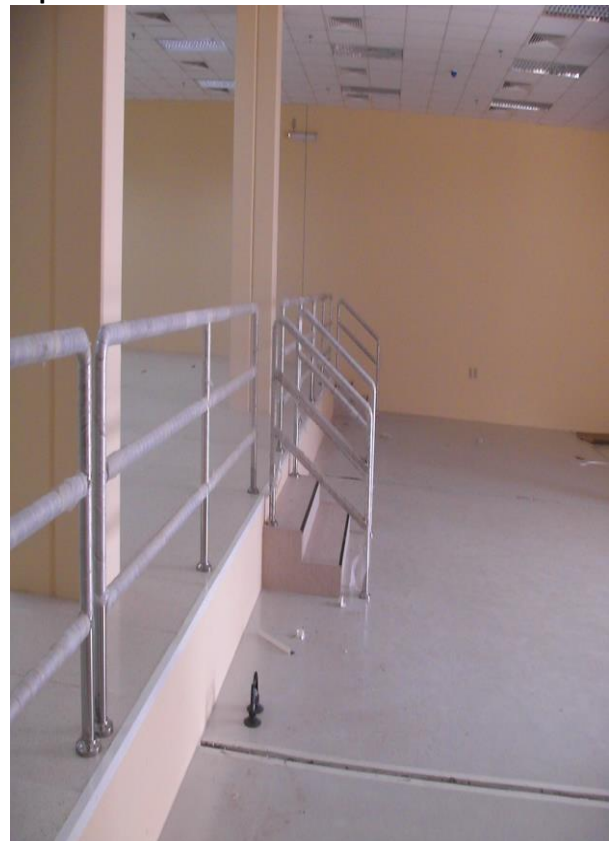
Raised floor system for Training Building
