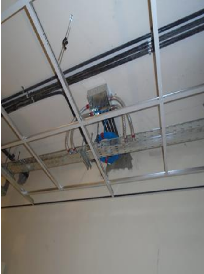
Cabling work, Eskan Village, Riyadh
