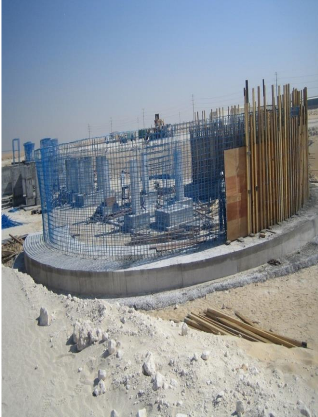
Foundation work for Steel Recycling Plant
