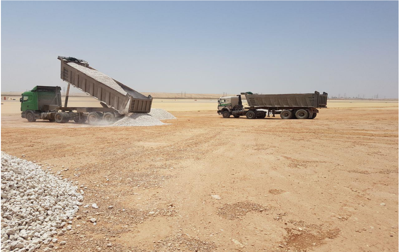
Supply and installation of Crushed Aggregate, Airfield-KAA, Riyadh
