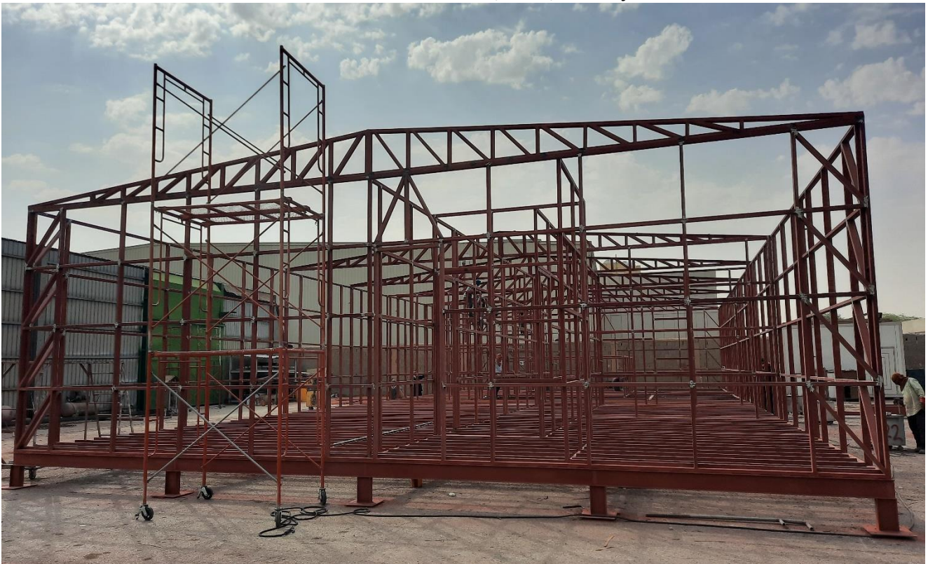
Fabrication of Administration Building (12m x 26m) at TDE Workshop - PSAB, Al Kharj-KSA
