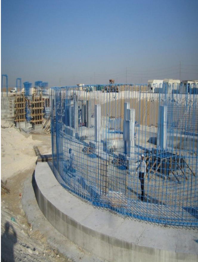
Foundation for Revolving Conveyor
