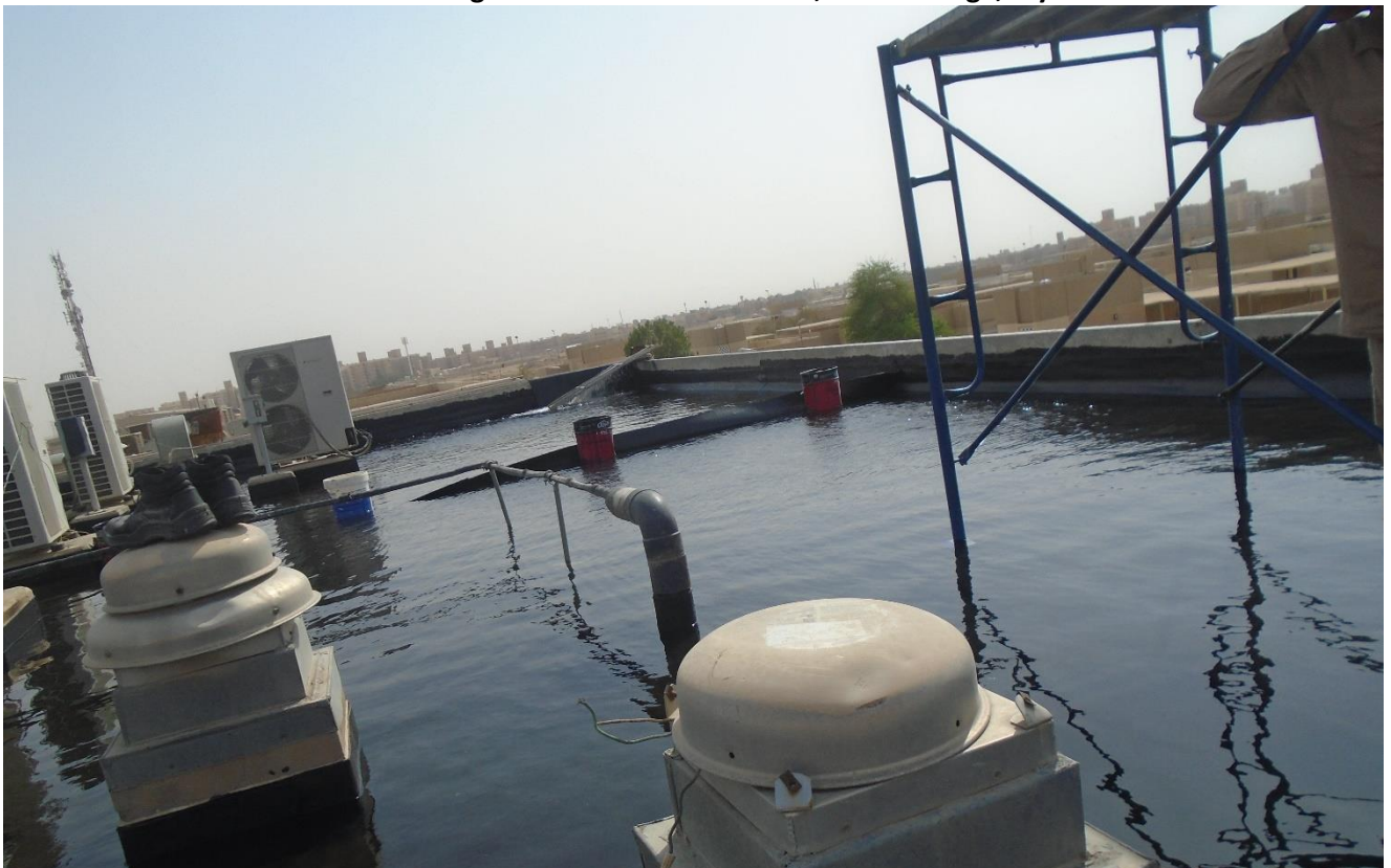
Waterproofing Test - Office Villas, Eskin Village, Riyadh
