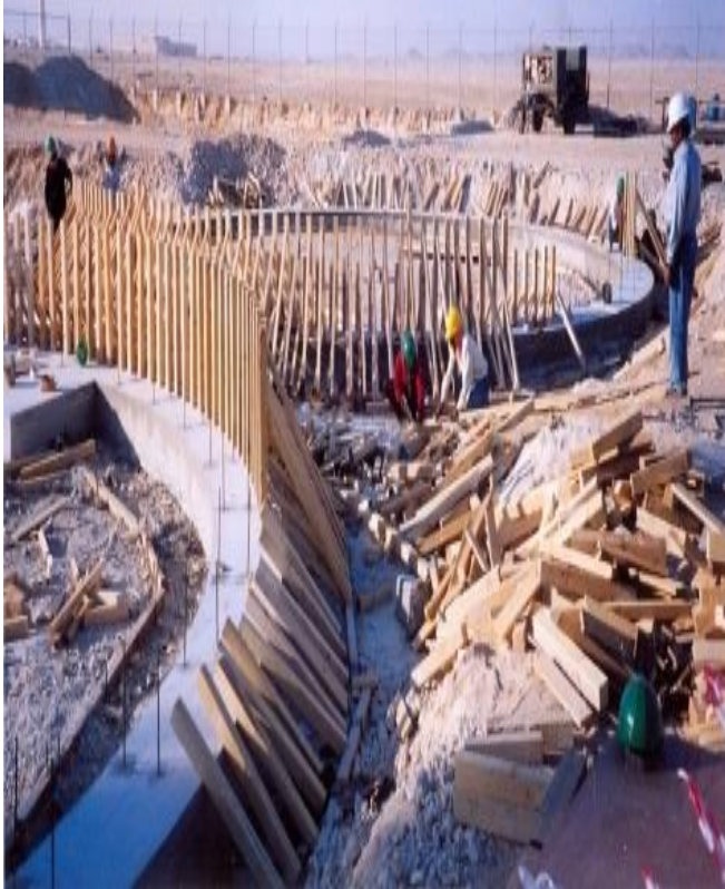
Form work for Metallic Tank foundations in Progress
