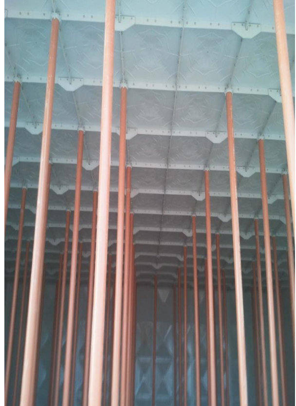
Erection of 1000M3 capacity water tank for fire suppression system
