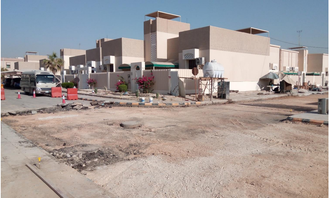
Road Construction – Eskan Village, Riyadh
