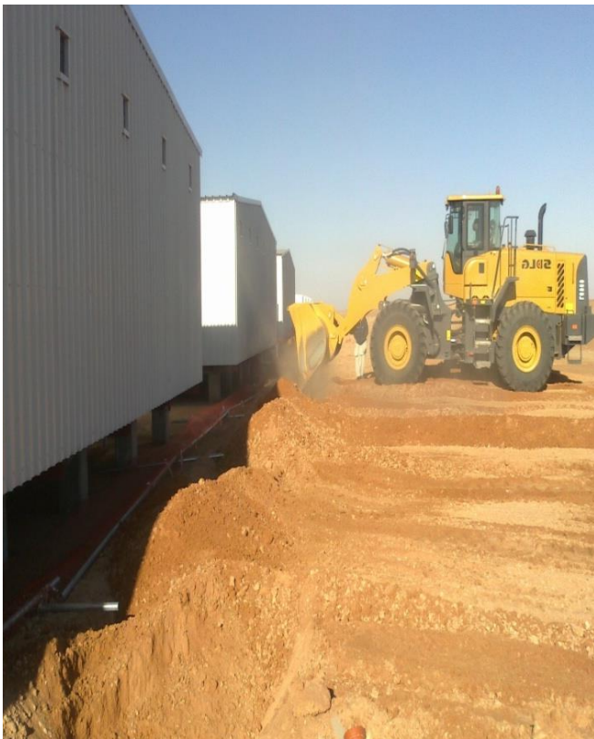
Utility Lines Backfilling
