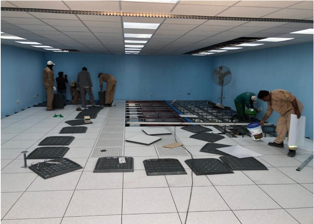
Installation of Raised Floor System and Perforated Tiles, NCC Trailer Building, PSAB, Al Kharj-KSA
