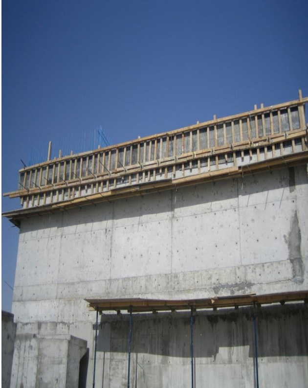
Multi Story Concrete Structure
