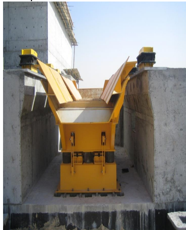
Installation of heavy machinery
