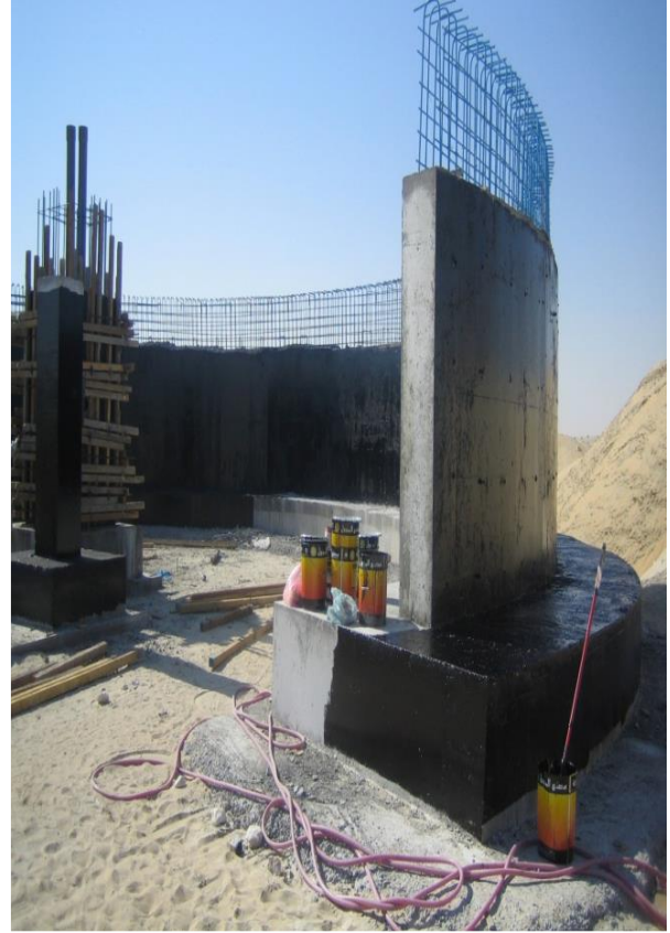
Revolving Conveyor foundation
