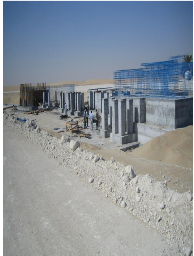
Foundation work for Steel Recycling Plant
