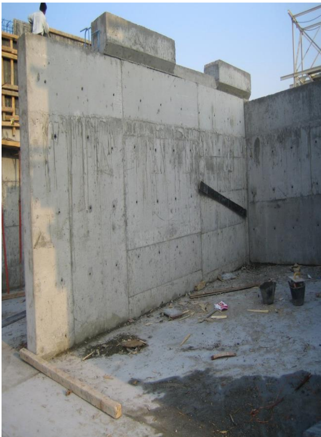
Concrete walls for Plant Base
