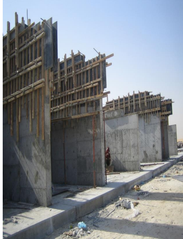
RCC walls for Product Storage area. Re-cycling Plant
