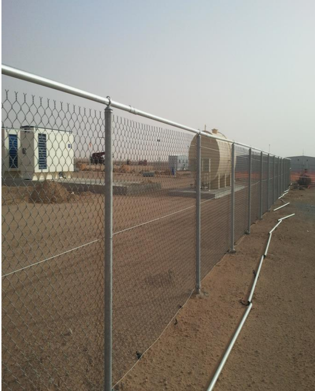
Chainlink fence Installation
