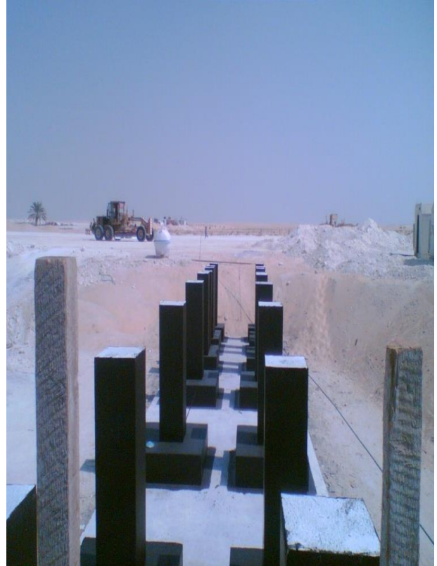
Foundation work for Steel Recycling Plant
