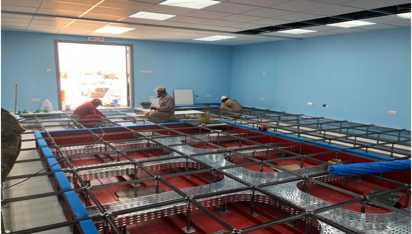
Instalaltion of Cable Trays, NCC Trailer Building, PSAB, Al Kharj-KSA
