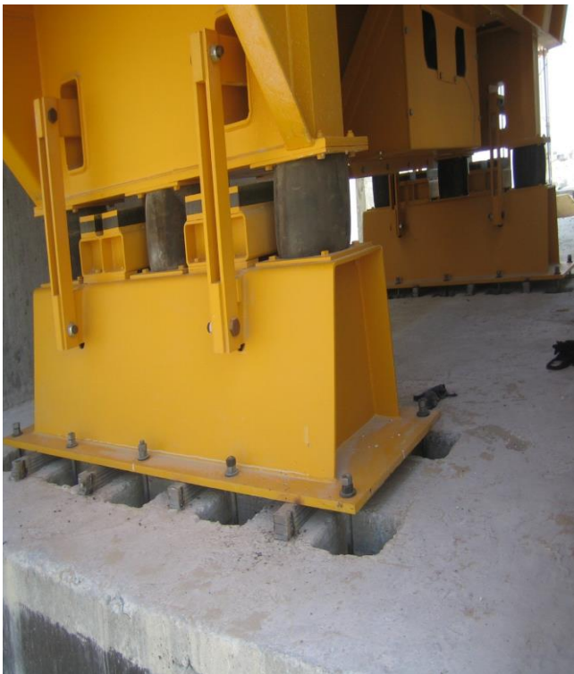
Installation of heavy machinery
