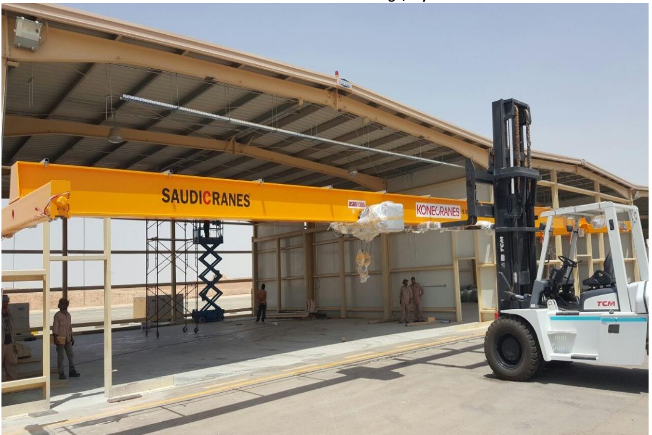
Instalaltion of Overhead Crane, Modification of Heliport Sunshade Project, KAA, Riyadh-KSA
