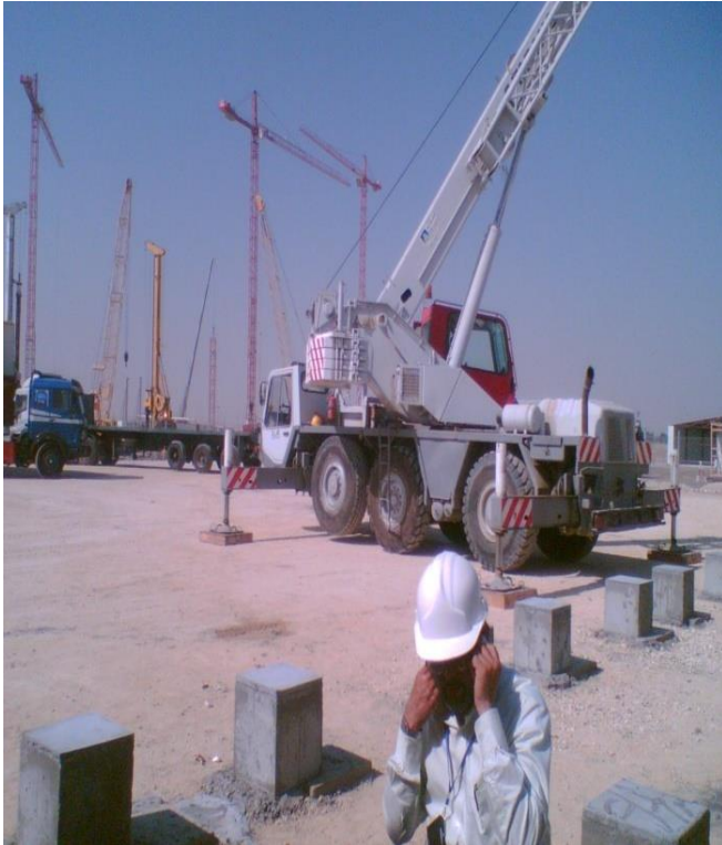
Portacabin Foundation works Temporary facilities
