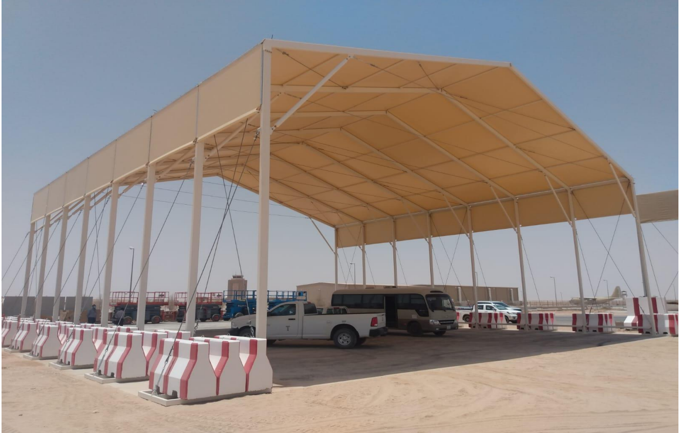
Equipment Sunshade, PSAB, Al Kharj-KSA
