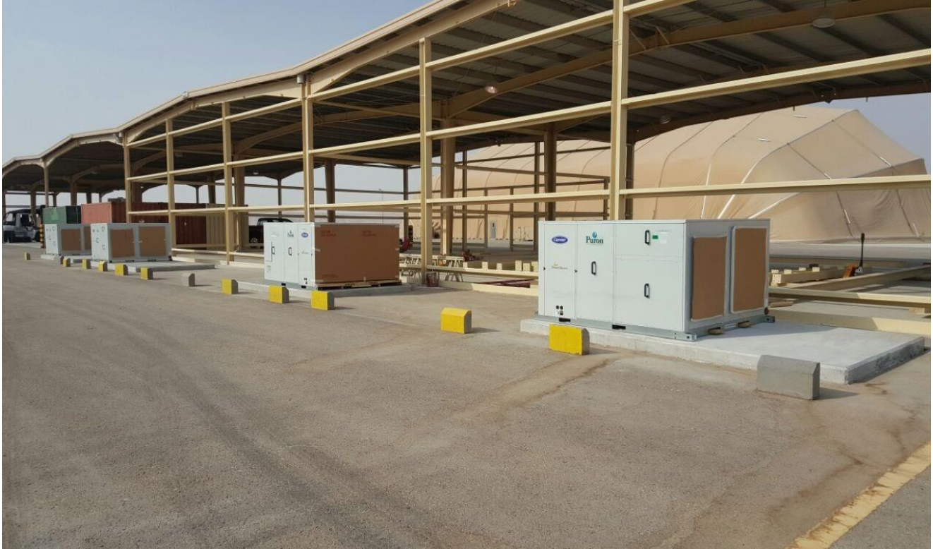
Construction of Heliport Sunshades, KAA, Riyadh-KSA
