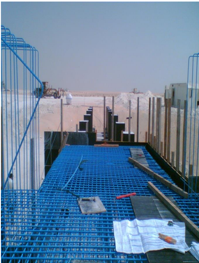
Foundation work for Steel Recycling Plant
