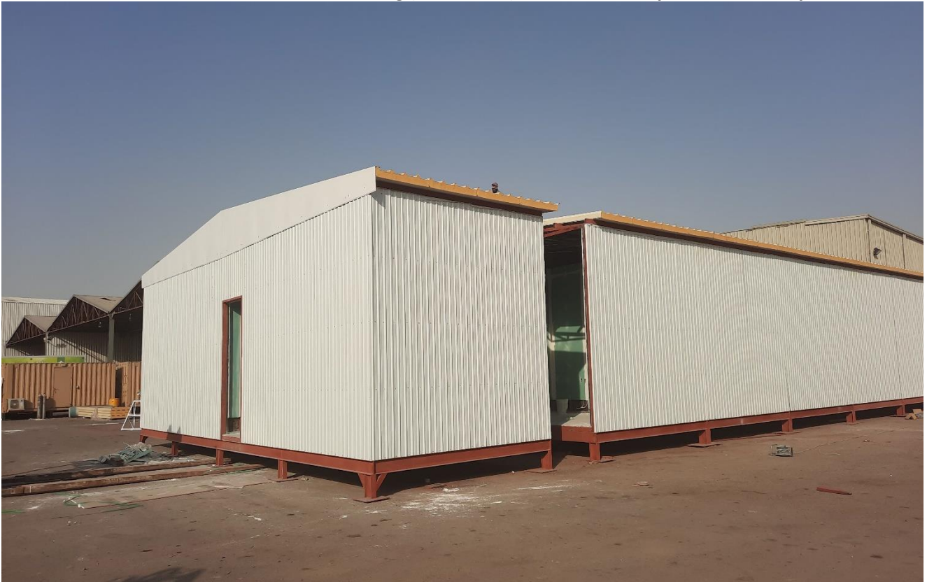
Fabrication of Administration Building (12m x 26m) at TDE Workshop - PSAB, Al Kharj-KSA
