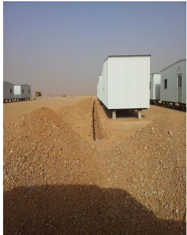
Ma'aden Main Camp Buildings being installed and trenching for sewer lines
