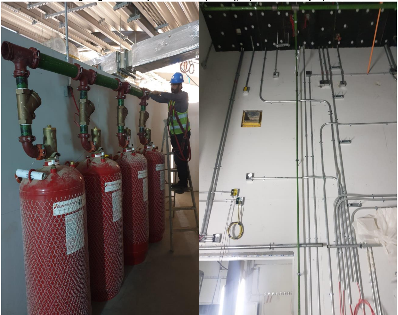
Fire Fighting and Fire Suppression Work (FM200), Riyadh Metro Project, KSA
