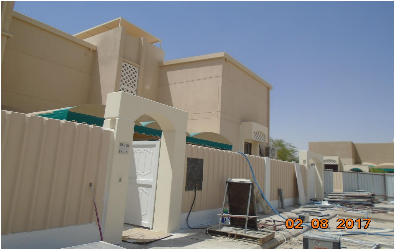
Renovation of Residential Villas – Eskan Village Riyadh
